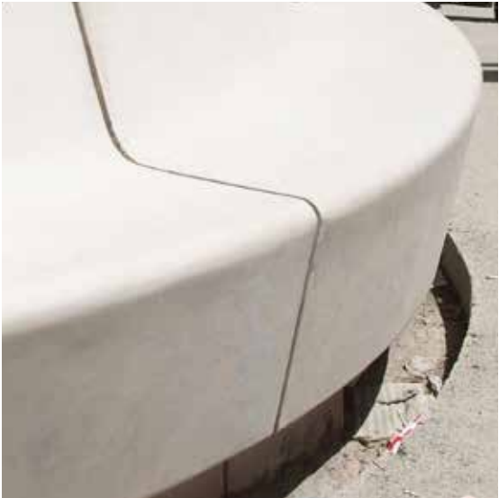
in situ concrete to achieve consistent bleacher curve
